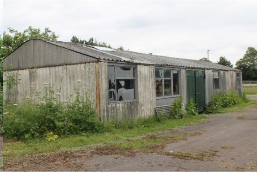
Existing building south facing.
